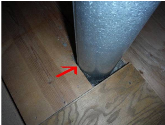
Vent pipe lacks proper clearance
