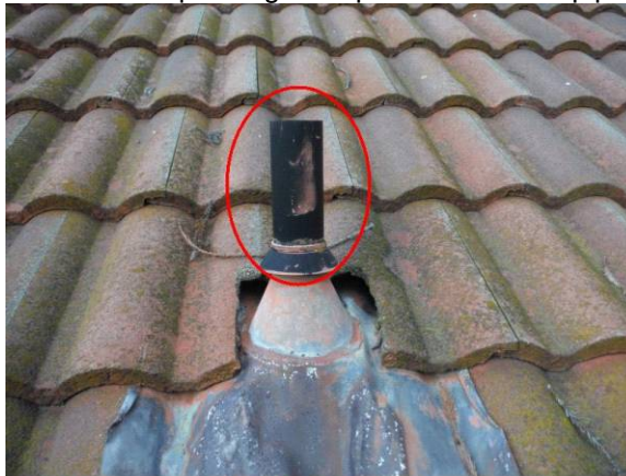
Paint exposed ABS vent pipes
