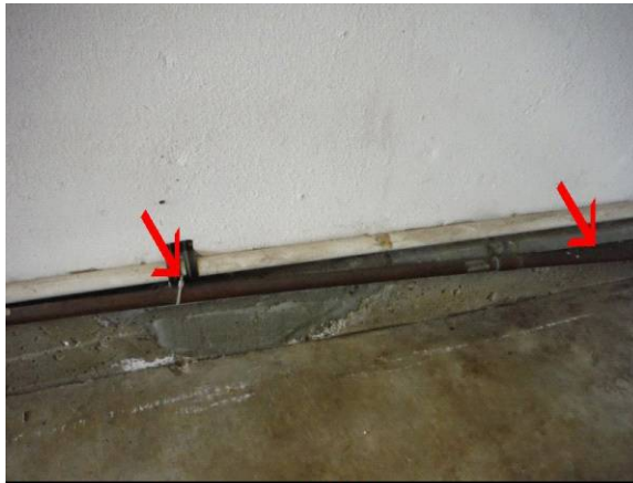
Improperly supported lines
