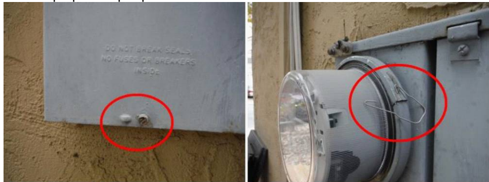
Missing and damage seals
