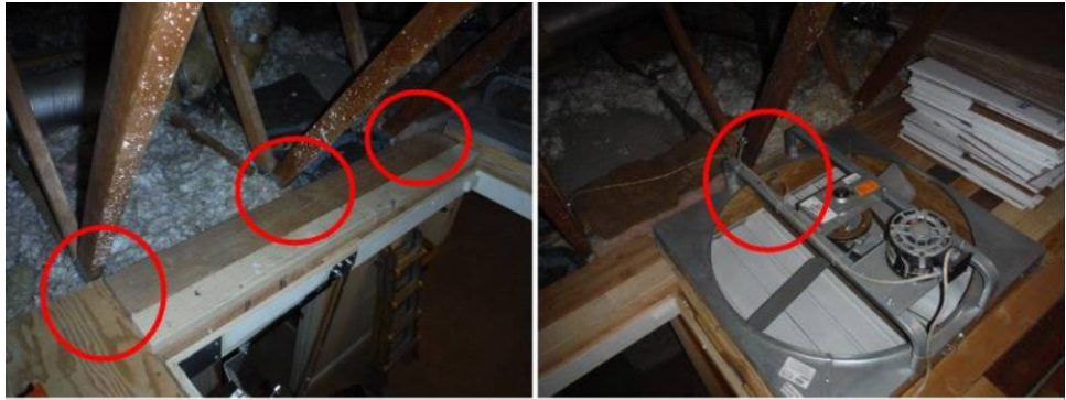
Altered truss framing
