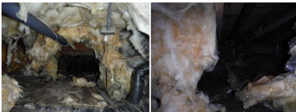
Loose/damage insulation
